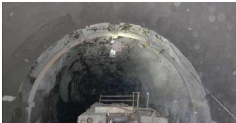
Fig. 14. Application diagram of the U-shaped steel support
