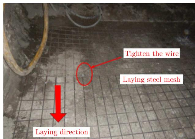
Fig. 8. Laying reinforced mesh
