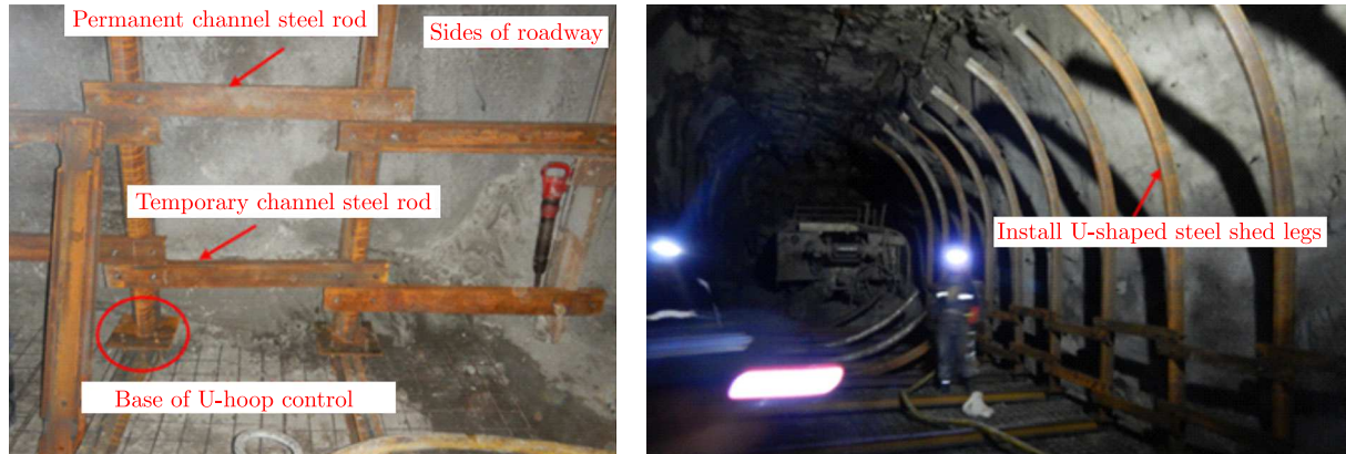
Fig. 9. Field installation of U-shaped steel shed legs
