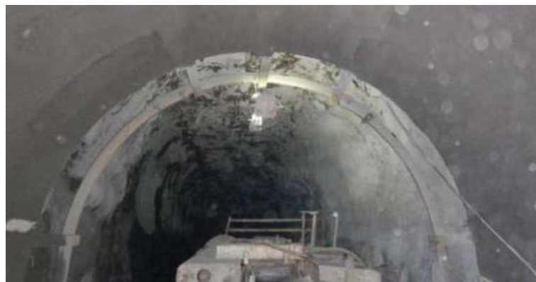
Fig. 14. Application diagram of the U-shaped steel support
