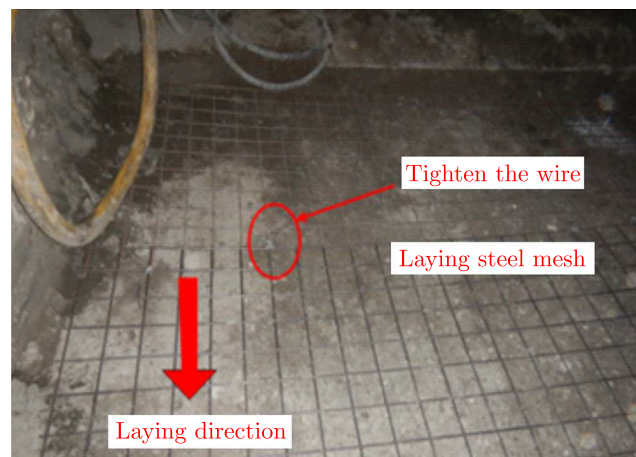
Fig. 8. Laying reinforced mesh
